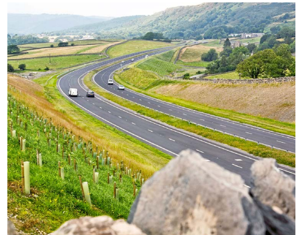
Image 1.2 Stone walls, and earthworks recently planted with woodland to integrate the A590 in Cumbria into its landscape context
